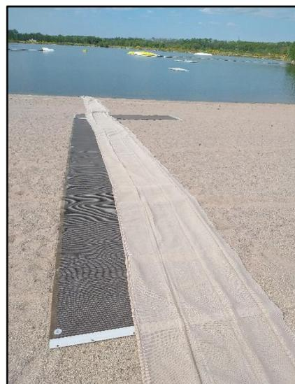
**Step 2:** Install the first spike in the end sock and anchor it vertically. The top of the Sandfence and the spike must be at most 1m from the ground.
